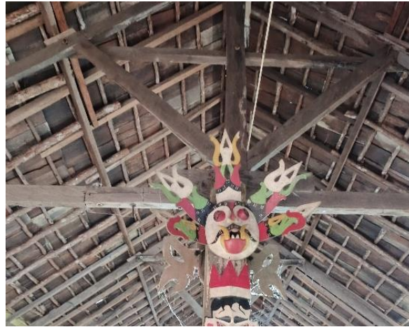
Figure 2. Roof of the Betang Hapakat House (Wooden Shingles)
