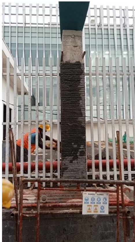
Picture 5. Application product rock natural Dhafin Stone as material wall on project construction (Source: Dhafin Stone Documentation, 2026)
