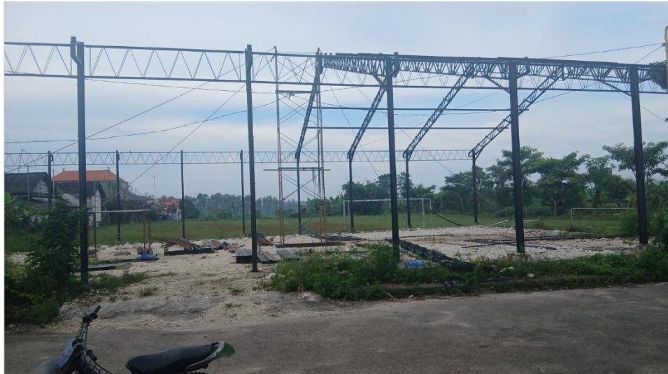
Figure 1. Field conditions in Lembor Village during the construction of the red and white village cooperative
