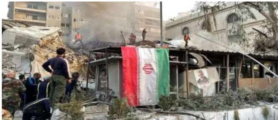
Figure 1. Condition of the Iranian Consulate Building in Damascus after the Israeli Airstrike on April 1, 2024
